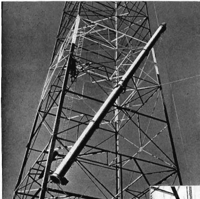
Raising the four-section Pylon in one completely assembled unit at WJPG-FM, Green Bay, Wisc.
